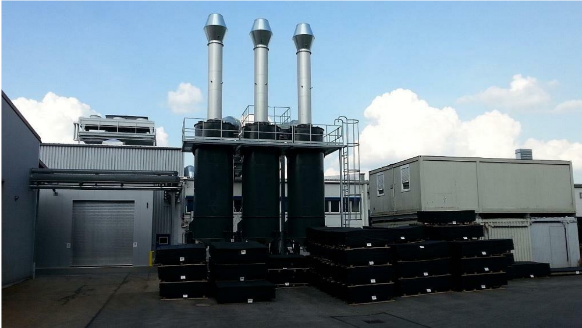
Carbon modules as final stage for gas and odour ashes removal. (Fig.: KMA)
