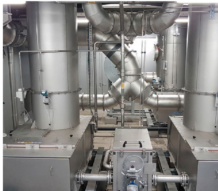
The moisture is removed from the cocoa nibs in the large roasting drum. Right: The three KMA gas scrubbers cool, humidify and clean the cocoa exhaust air in preparation for the biofilter.
